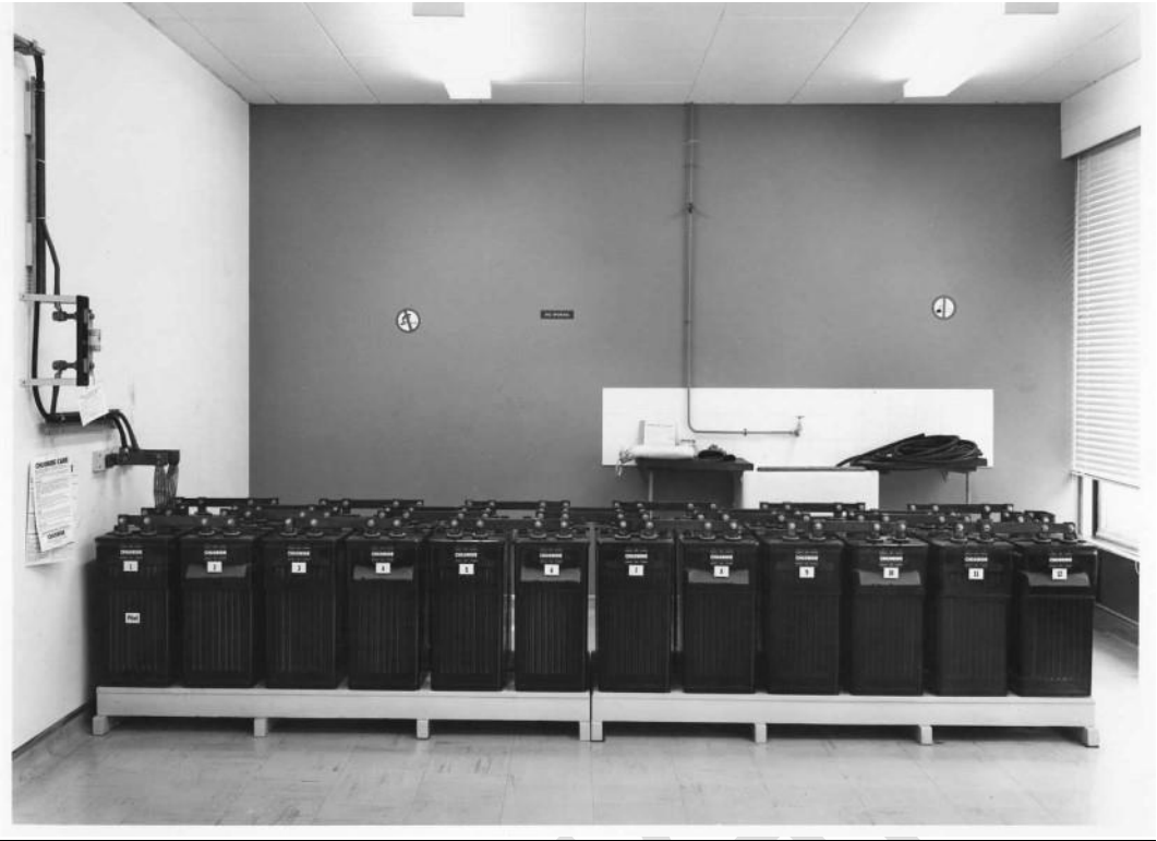
Fig 13 'Emergency Power Supply, P.B.X. Room'
